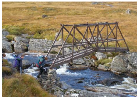
The wire-stayed bridge over the Alder Burn, near Ben Alder Cottage
